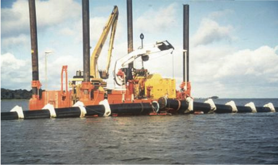
Fig. 1. Launch of a submerged pipe with junction in the sea.
