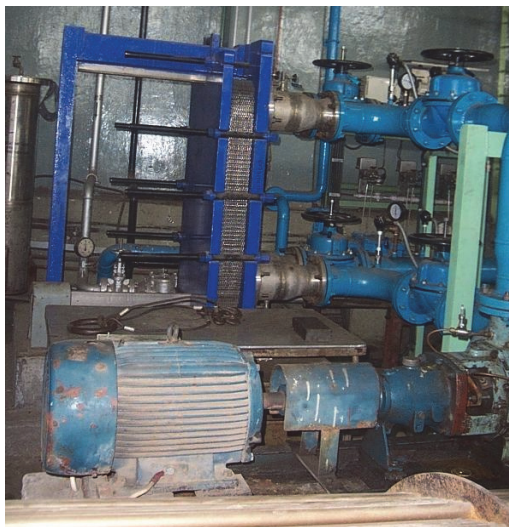
Fig. 1. Plate type H.Ex to transfer heat from primary coolant to intermediate circuit.
